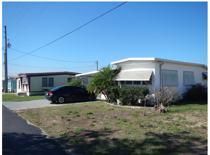
8PO08219_l Facing Southwest
