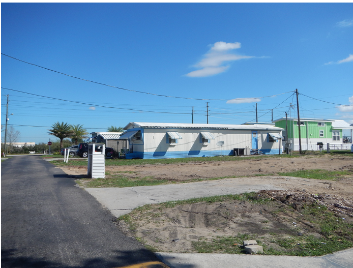
8PO08219_k Facing Northeast
