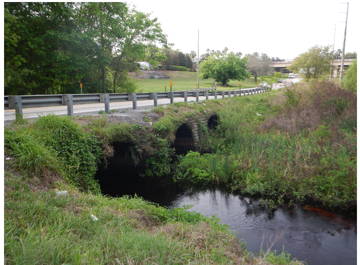
8OS03232_d Facing South
