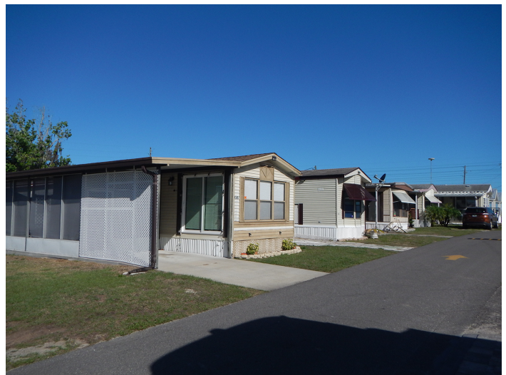
8PO08219_d Facing North
