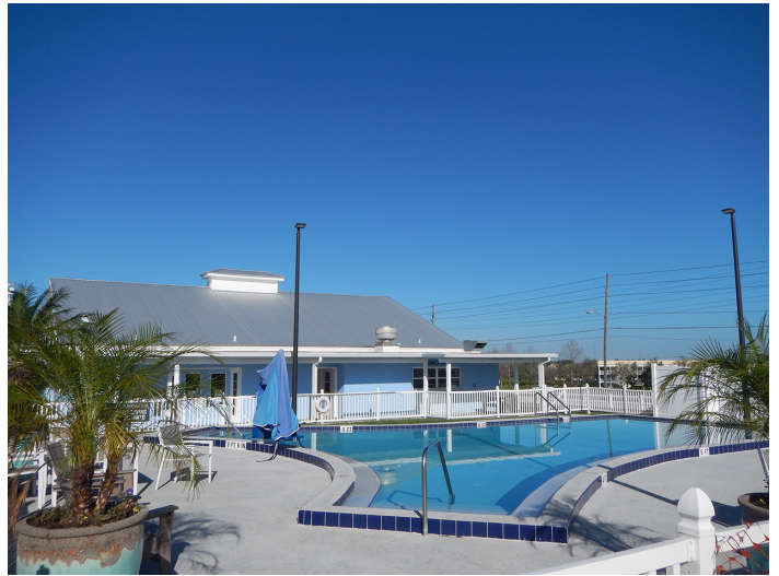
8PO08220_b Facing Northwest
