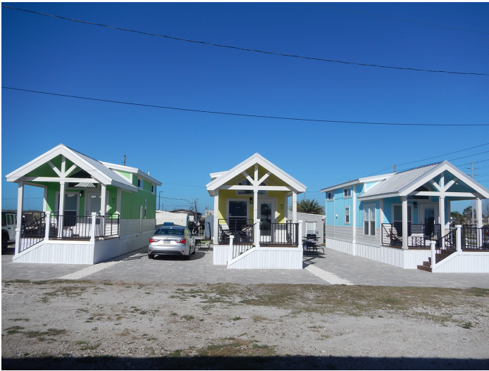
8PO08219_a Facing Southwest
