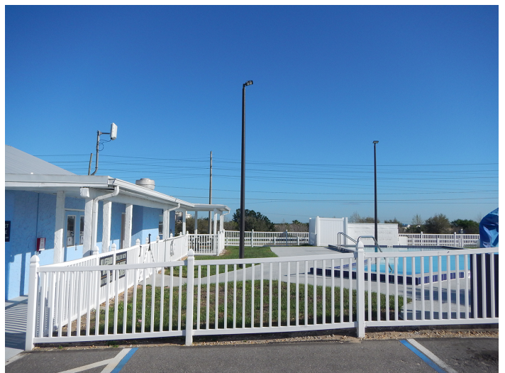
8PO08220_f Facing North
