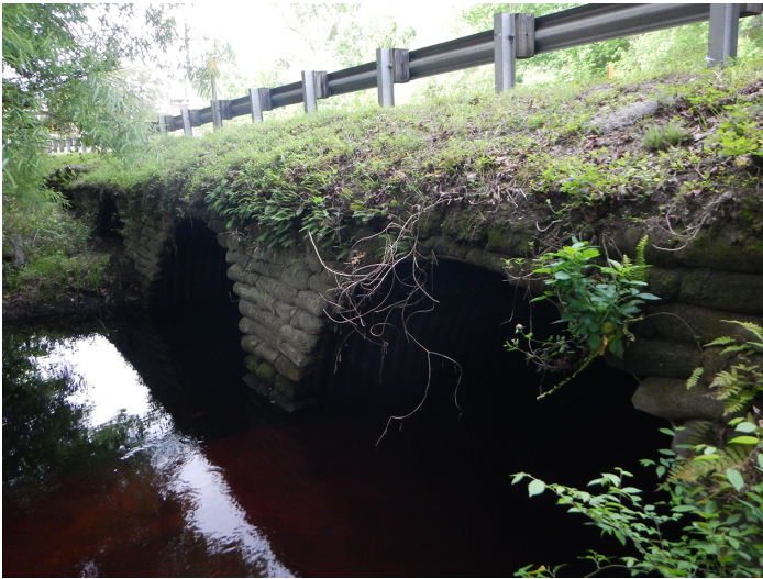
8OS03232_a Facing Northeast
