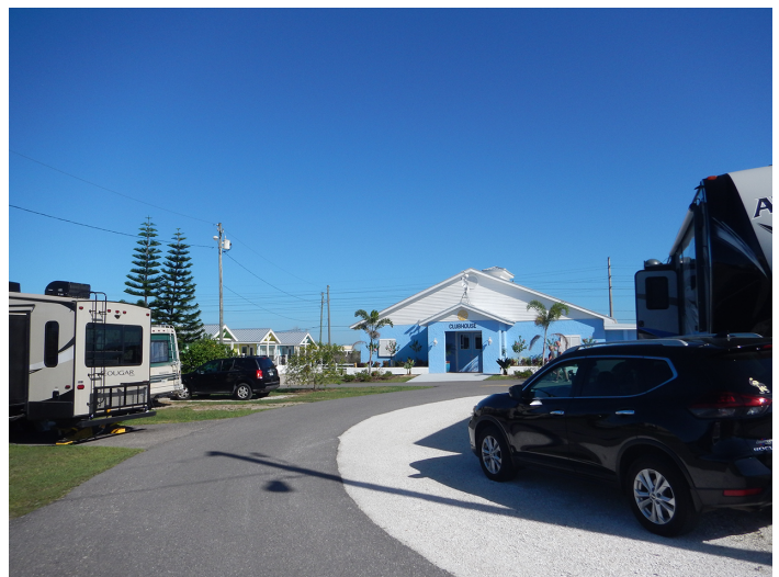
8PO08219_f Facing North
